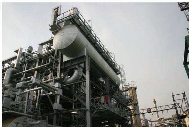
Figure 3. The new sulfur plant in Gelsenleirchen-Horst refinery with two Claus reactors and an LT-SCOT reactor in one shell.
